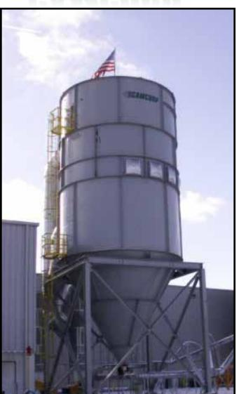
**CAMCORP** offers two style of reverse air collectors. The HVP (High Volume Pulse) collectors utilize a rotary lobe blower as the cleaning energy to pulse the bags clean. The SWF (Sweep Arm Filter) utilizes a high static fan to clean the bags. Both have a rotating arm within the clean air plenum to deliver the cleaning air.
